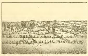
TWIG FENCING FOR FIXING LOOSE SAND
